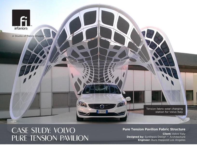
The "PURE Tension" Volvo Pavilion was a collaborative effort between Fabric Images®, Synthesis Design + Architecture (SDA), and Buro Happold (BH). The design began as a concept, commissioned by Volvo Car Italia to showcase the new Volvo V60 Plug-in Hybrid. The purpose was to create a lightweight, rapidly deployable, tensioned membrane structure that would act as a portable charging station, fitting within the car's trunk.
